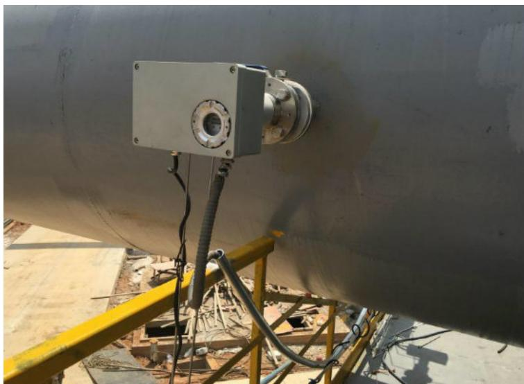
**KF series Laser Gas Analyzer** developed aiming at the industrial on-line analyzing, environmental on-line monitoring. Many types of the KF series Laser Gas Analyzer are available, including in-situ probe, by - pass type, multi-channel and Disc mounted type etc. Gas types like O<sub>2</sub>, CO, NH<sub>3</sub>, CO<sub>2</sub>, CH<sub>4</sub>, H<sub>2</sub>O HC, HF etc. can be analyzed. The concentration analyzing of target gases contains the macro-analysis and micro-analysis.
