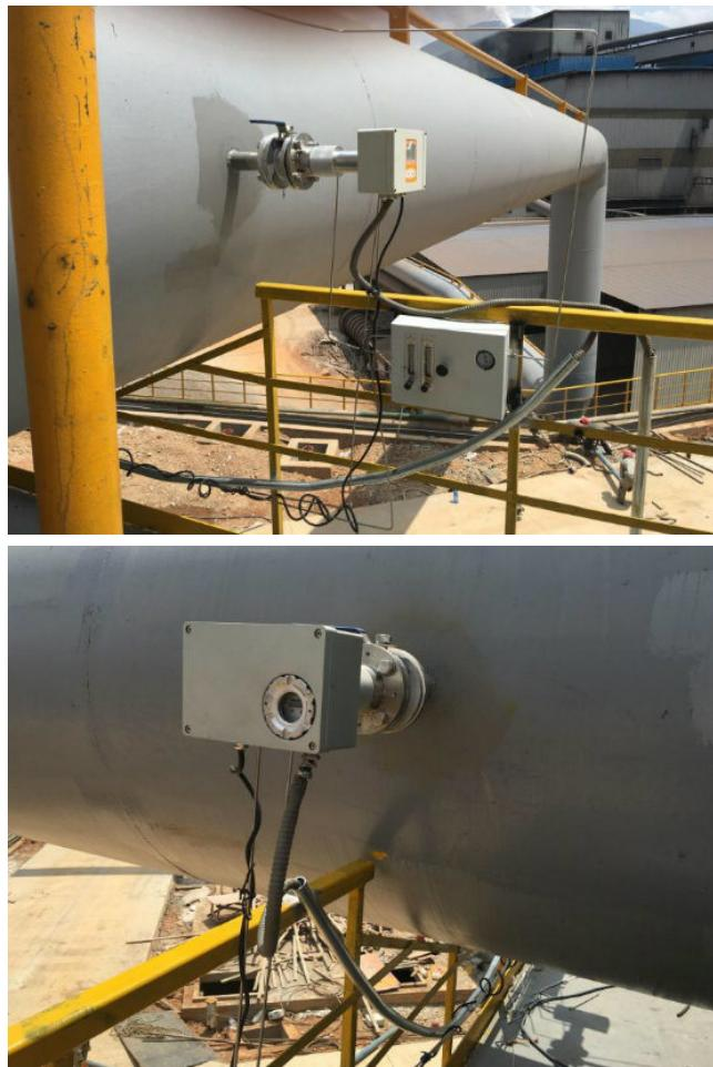
The KF series Laser Gas Analyzer is developed for industrial online analysis and environmental online monitoring applications. Multiple configurations are available including in-situ probe, bypass type, multi-channel, and disc-mounted types. The analyzer detects various gas types including O<sub>2</sub>, CO, NH<sub>3</sub>, CO<sub>2</sub>, CH<sub>4</sub>, H<sub>2</sub>O, HC, HF and others, with capabilities for both macro-analysis and micro-analysis concentration measurements.
