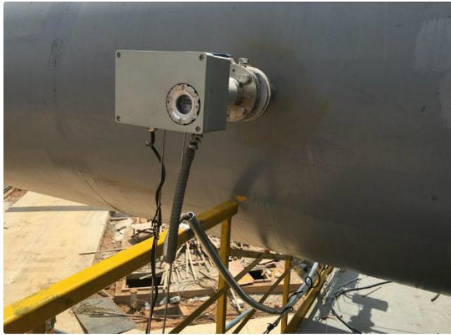
The KF series Laser Gas Analyzer is developed for industrial online analysis and environmental online monitoring. Available in multiple configurations including in-situ probe, by-pass type, multi-channel, and disc-mounted types. Capable of analyzing gases including O<sub>2</sub>, CO, NH<sub>3</sub>, CO<sub>2</sub>, CH<sub>4</sub>, H<sub>2</sub>O, HC, HF and others, with both macro and micro concentration analysis capabilities.
